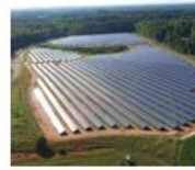
Cypress Creek solar farm, Massachusetts
